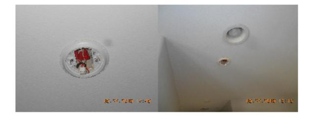
One or more of the smoke detectors have been removed. We recommend installation of smoke detectors in compliance with todays standards.
