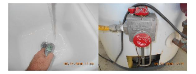
The temperature is set too high. Excessive temperature can be dangerous and inefficient. We recommend the temperature setting be lowered to provide safer, more efficient operation.
