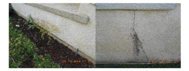
There are moderate sized cracks in the stucco that should be patched and sealed as part of preparation for the next painting. Flexible patching materials are recommended rather than rigid cementious patching compounds.
